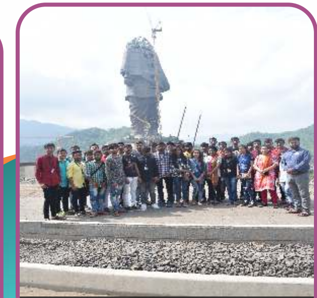
"Work has been completed upto full body"
